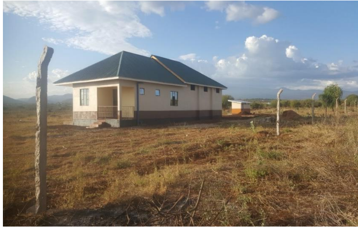
Guard House + Supplies store (completed in June, 2019)
