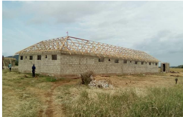
The proposed 20 room Children's Home (In progress since late July, 2019)
