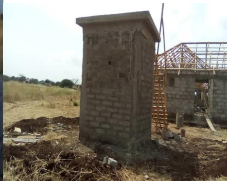
Constructing water tank tower (June, 2019)
